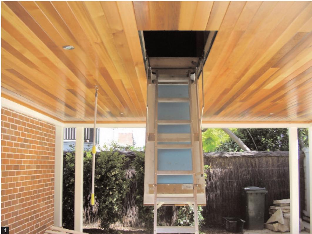
1. Ultimate series fitted to double carport, timber paneling is also fixed to hatch door to provide a consistent finish to the ceiling. This provided access for the owner into area over the garage as well as the carport.
