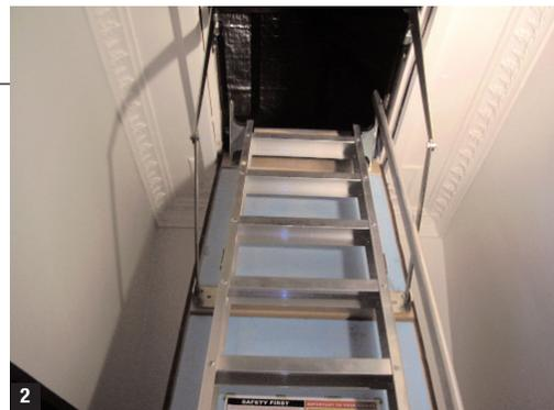
insulated door, a door seal to minimise drafts and dust, injection moulded non-slip EVA feet, and can be easily fitted with extra handrails to suit the client.
